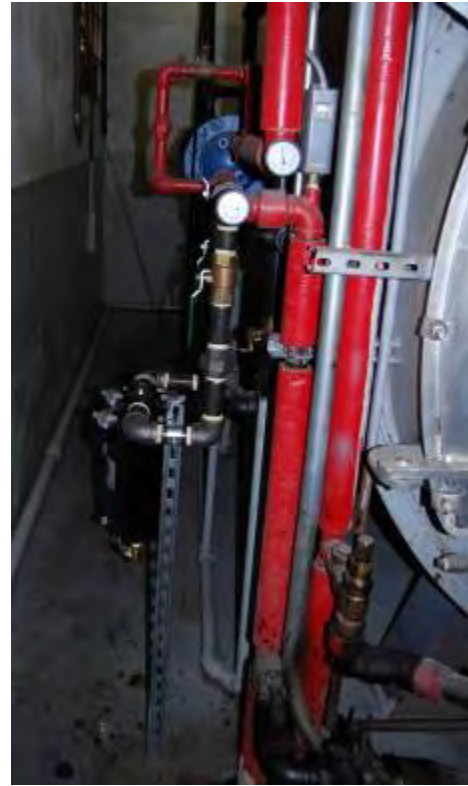
Fitch Installation on Boiler Fuel Line
